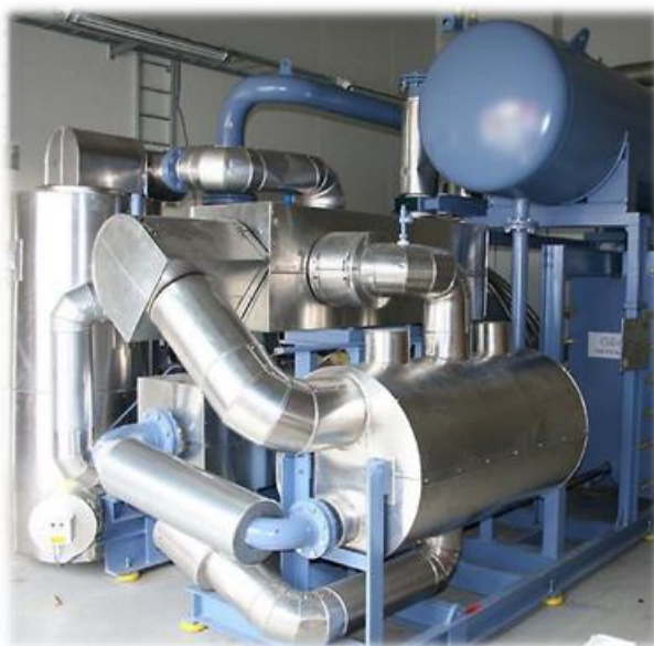
Figure I.3 Example – heat pump unit with ammonia/R717 (max. 82 °C)
