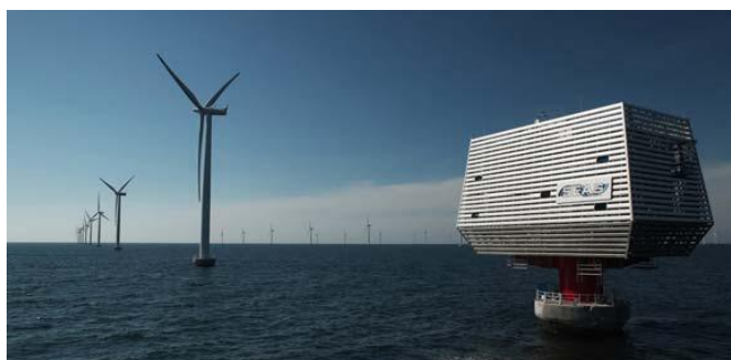
Figure 5-2 Nysted offshore wind farm offshore substation 58
