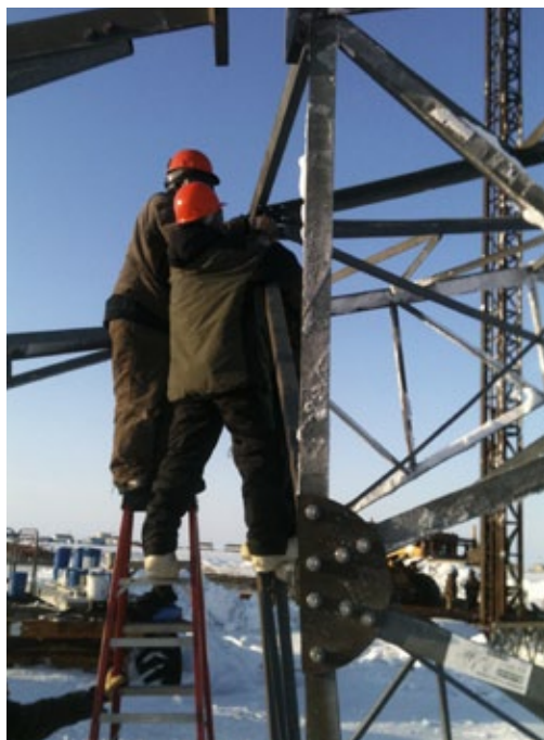
▼ Community members installing wind turbine towers
