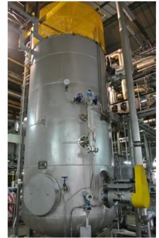
Electric boiler (steam)
