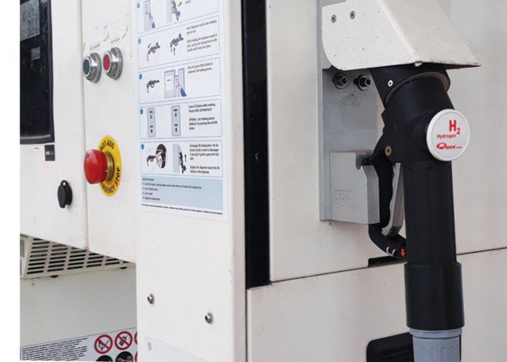
Hydrogen filling station for electric vehicles with fuel cells (Picture: Mats-Ola Larsson)
